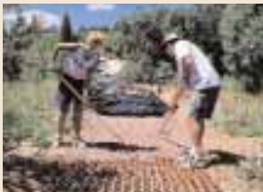
Covering with tarp to cure
