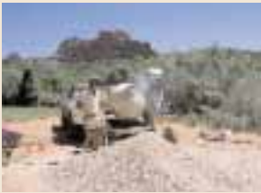
Tumbling in mixer— 1 / 2 "– 3 / 4 " gravel, 7% cement as binder, and terra cotta colorant to match native soils
