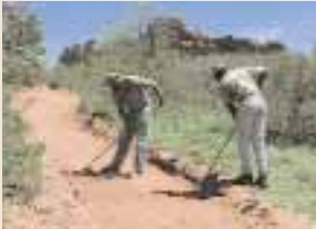
Trenches filled with base course, leveled and compacted
