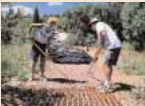
Covering with tarp to cure
