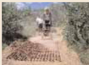
Compacting gravel mixture into Surefoot 4 mats and misting with water for adhesion
