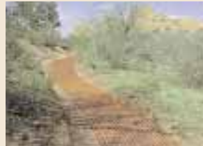
Shaping Surefoot 4 to curves and hills, and anchoring in place
