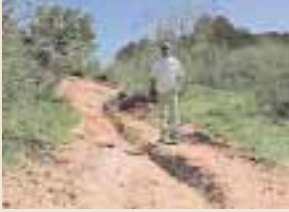
Rutting caused by horse traffic
